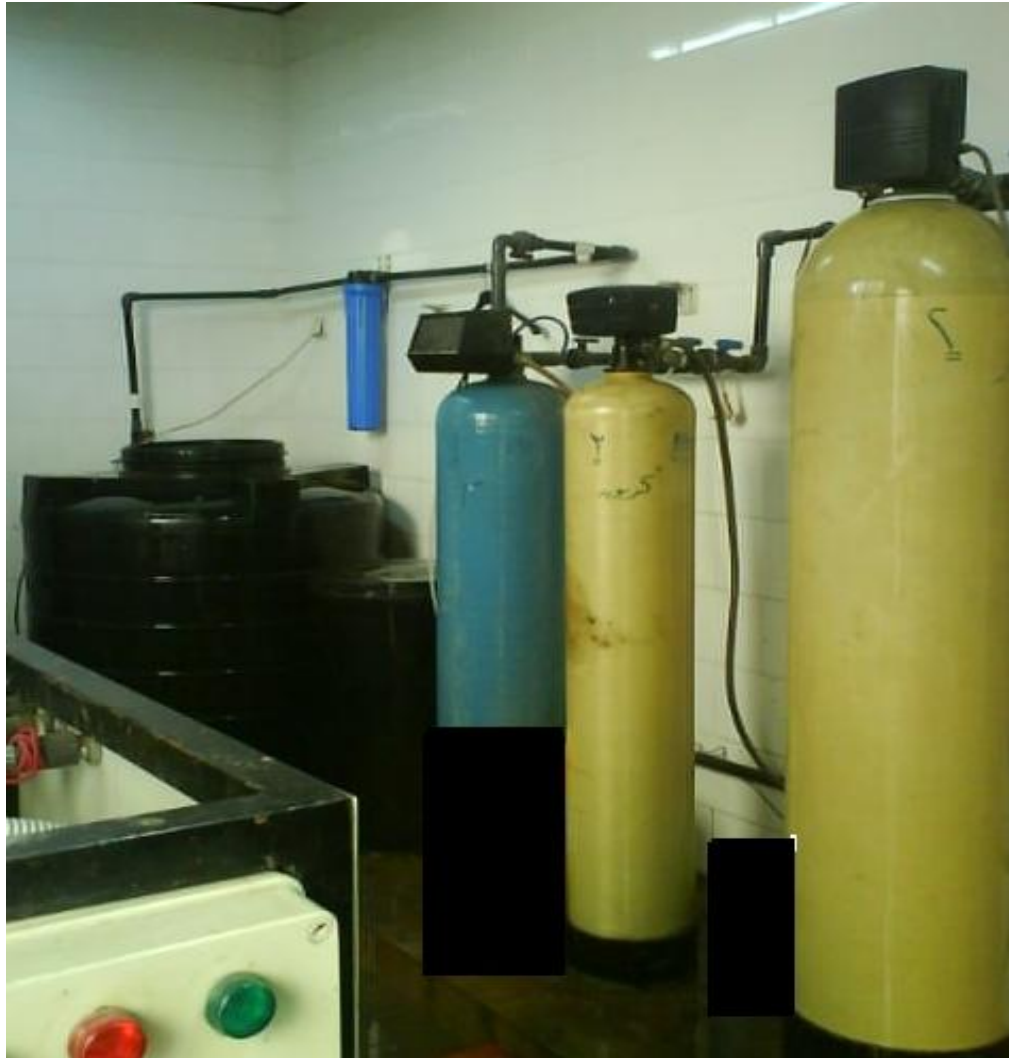
Community Purifying Unit (under construction)
