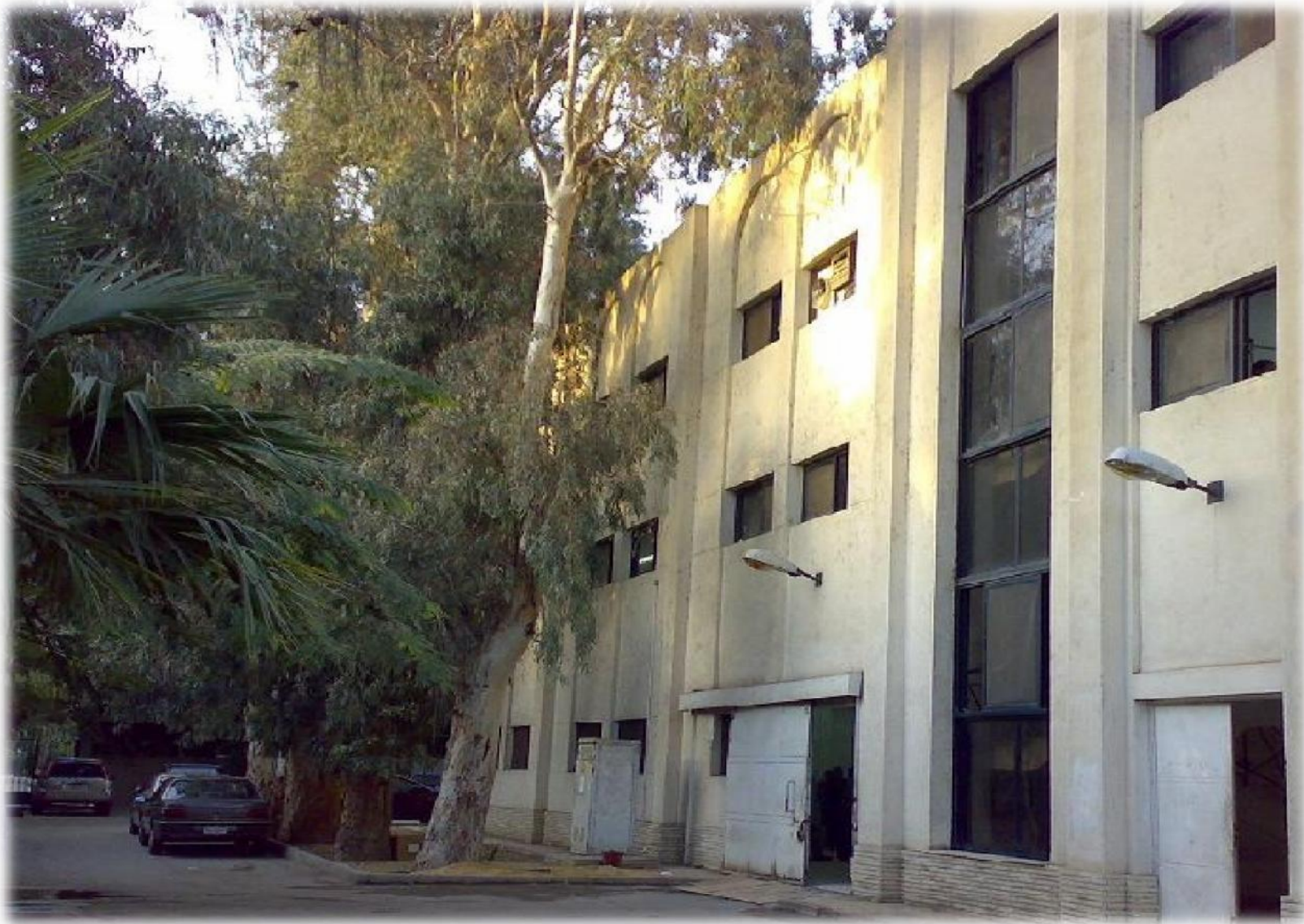
Factory Side View
